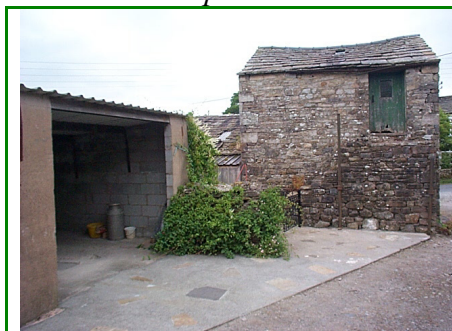
Garage & Barn store
